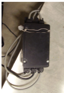
Junction boxes with wire security seals
